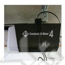
There are 3 wires of different color need to be connected to the back of the power head.
