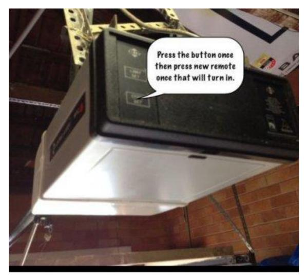
1. If you only have one motor, please program the top left button with the motor For the original remote, please set the SIDE BUTTON as UP and DIP SWITCHES AS FOLLOWING:
